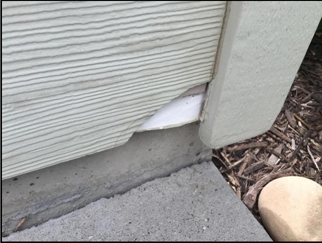
2.0 Item 2(Picture) Right of garage
